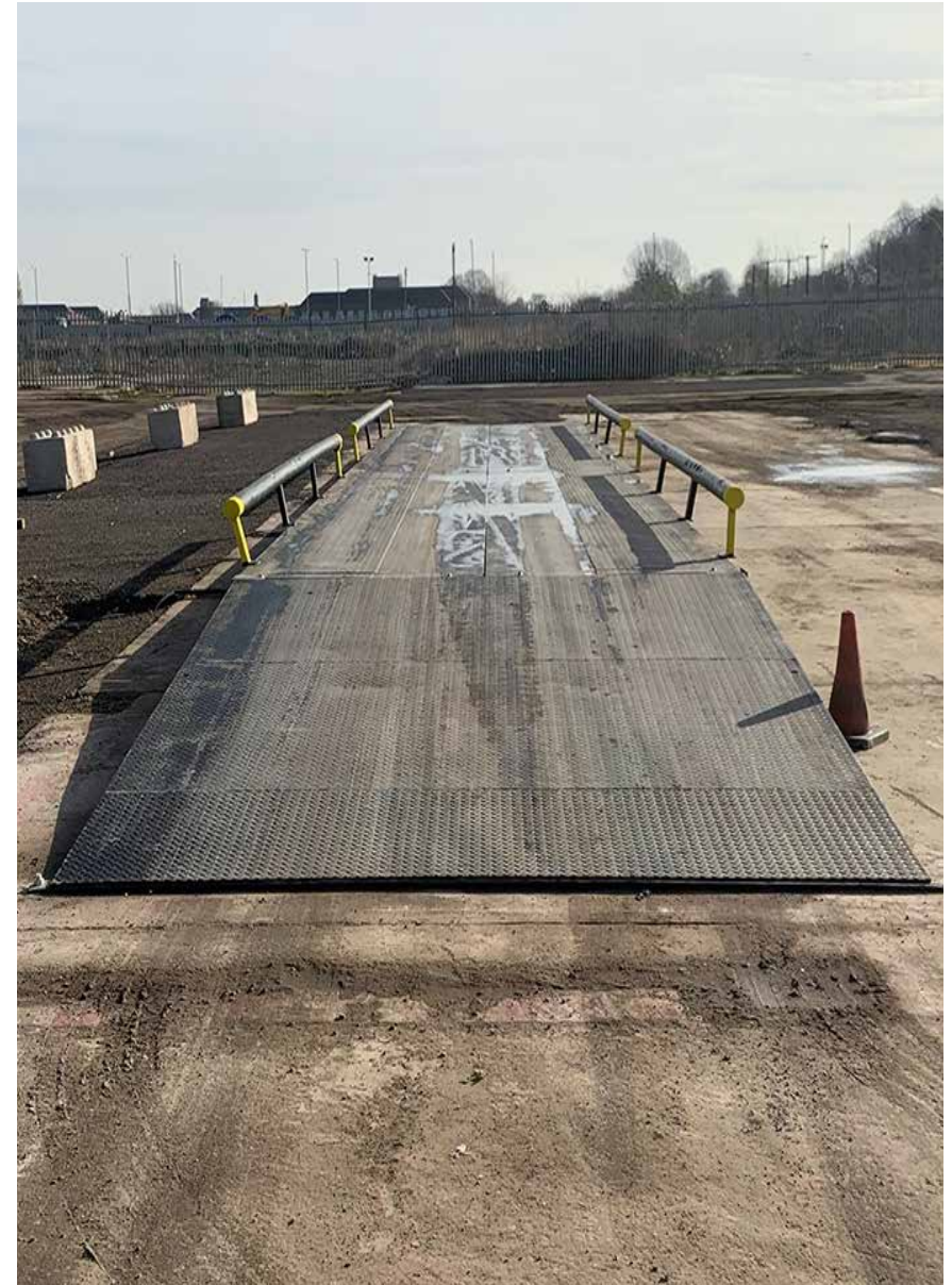
Project: Hire weighbridge installation at DGI Group, Chester Weighbridge: 15m x 3m Eco Deck with ramps
