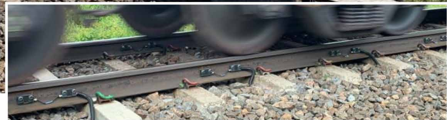
Picture 2 Same site during installation (sensors visible).
